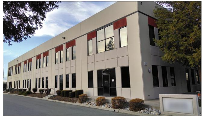
Figure 1-5. Concrete tilt-up wall building with wood light-frame roof diaphragm.
