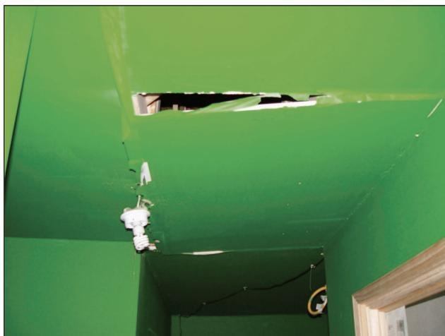
**Figure 4-2.** Ceiling diaphragm damage in two-story wood light-frame townhouse building that might be attributed to diaphragm deformation.
