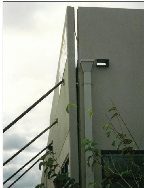
**Figure 4-1.** Concrete tilt-up building with wall connection to wood light-frame diaphragm damaged in the 1994 Northridge earthquake. External temporary braces have been added to stabilize the tilt-up wall.
