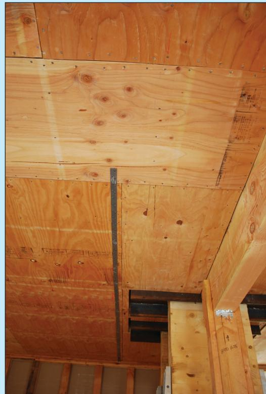
**Figure 4-4.** Detail of first floor diaphragm from Figure 4-3 test building, strengthened with plywood diaphragm sheathing, with collector strap applied over the face of the plywood sheathing.
