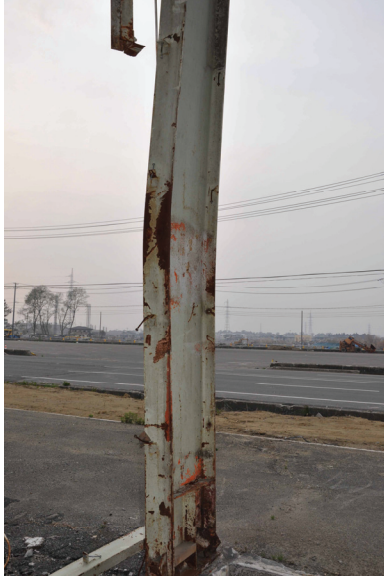
Figure A-12 Flexural buckling of a steel wide flange column (courtesy of D. Lignos).
