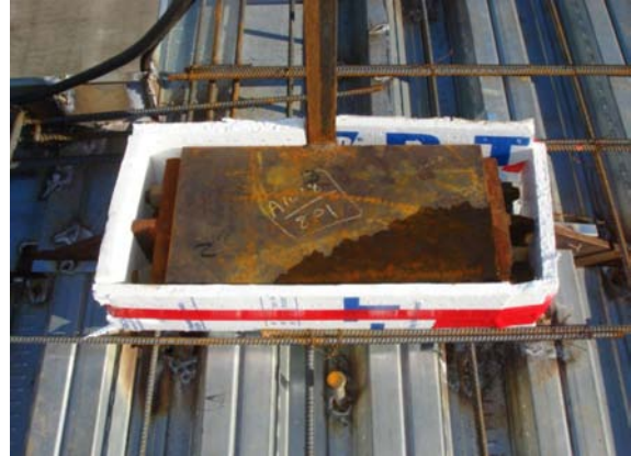
Figure 7-4 - Compressible material used to isolate a protruding bolted stiffened extended end plate connection prior to concrete placement.
