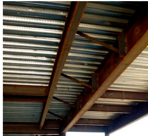
Figure 5-1 - Steel special moment frame beam stability bracing with a concrete filled metal floor deck.
