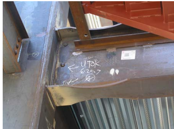
Figure 7-1 - Unauthorized attachment within the protected zone of a Reduced Beam Section connection.
