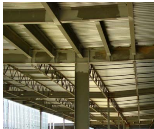
Figure 5-2 - Steel special moment frame beam stability bracing with a flexible unfilled metal roof deck.
