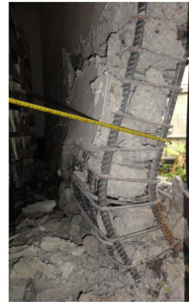
Figure 3-3 – Wall buckling, 2011 Christchurch earthquake.
