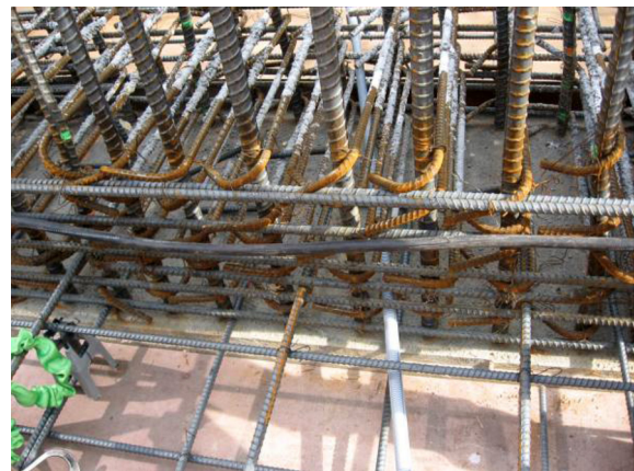
Figure 7-2 – Boundary confinement for planar wall.
