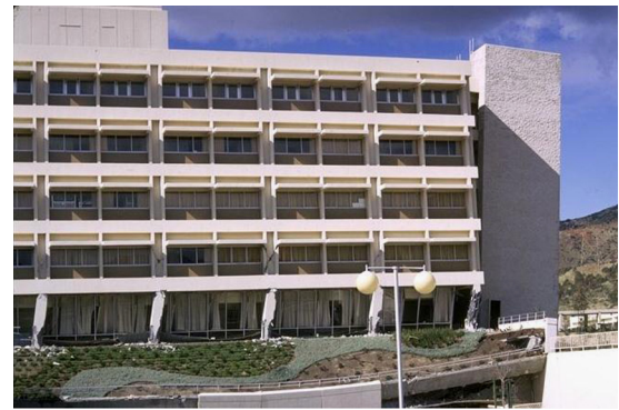
Figure 2-4 – Weak story damage, 1971 San Fernando earthquake.
