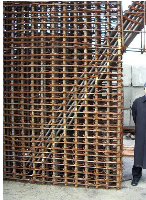
Figure 7-4 – Anchorage of diagonal reinforcement in heavily reinforced boundary element.
