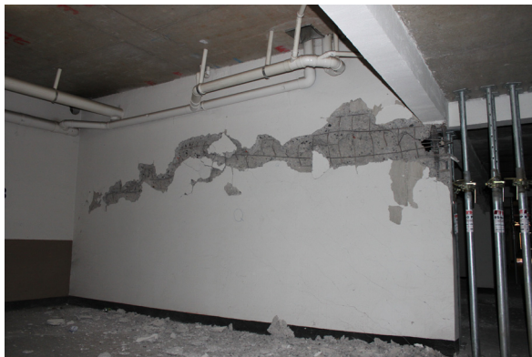
Figure 3-2 – Concrete crushing and reinforcement buckling of inadequately confined wall, 2010 Chile earthquake.
