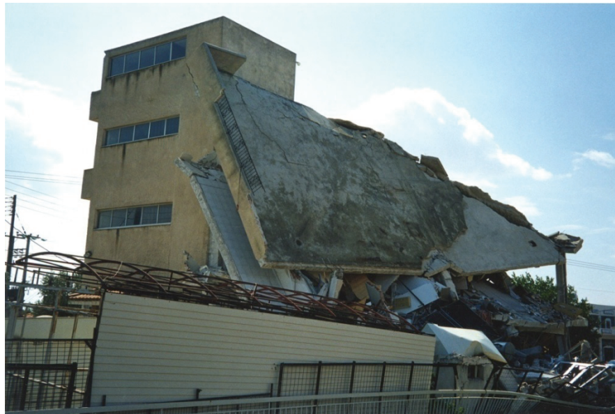
Figure 4-9 Collapse due to torsional drift demands in the 1999 Athens (Greece) Earthquake (Courtesy of NISEE Earthquake Engineering Online Archive).
