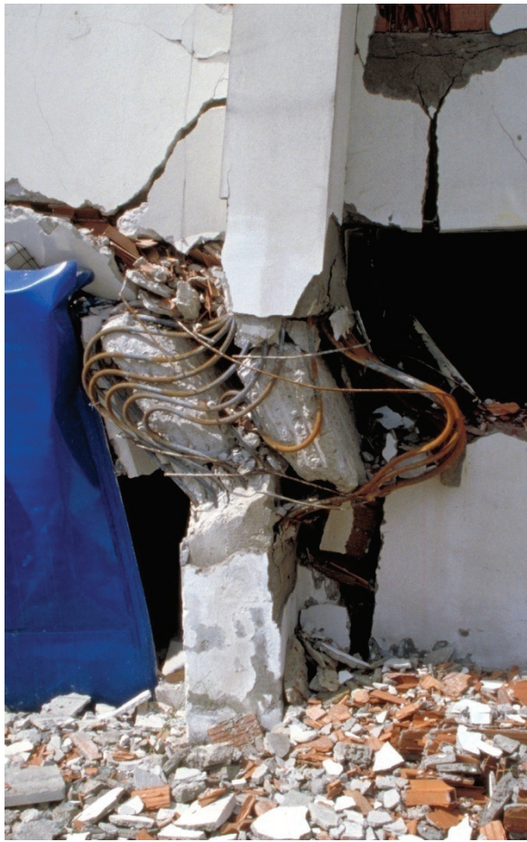
Figure 4-2 Column shear and axial failure in the 1999 Koceali (Turkey) Earthquake (Courtesy of NISEE Earthquake Engineering Online Archive).
