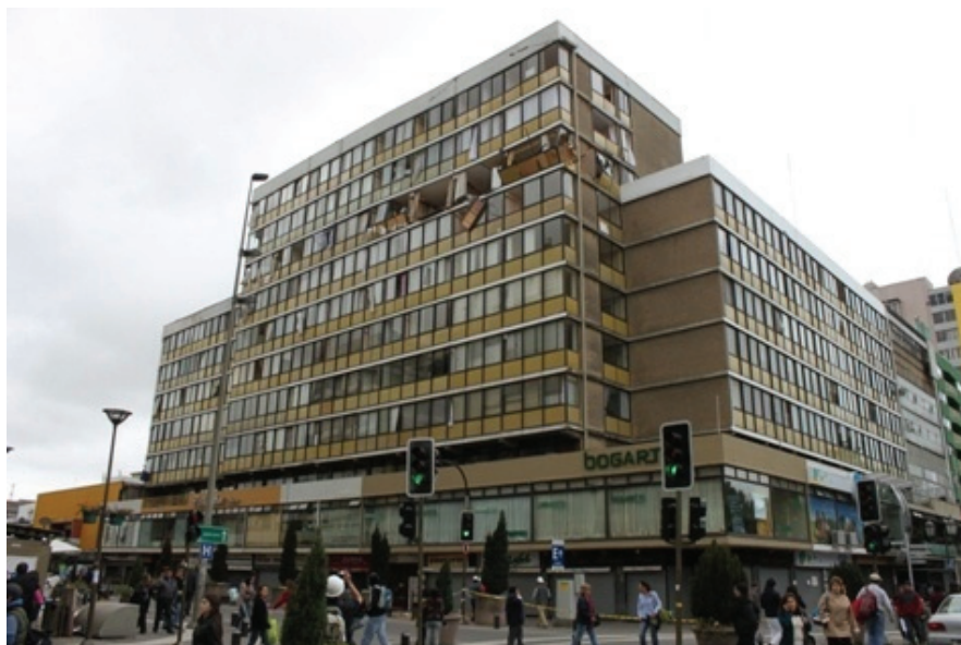
Figure 4-10 Story damage due to vertical irregularity, 2010 Maule (Chile) Earthquake (Courtesy of Jack Moehle).
