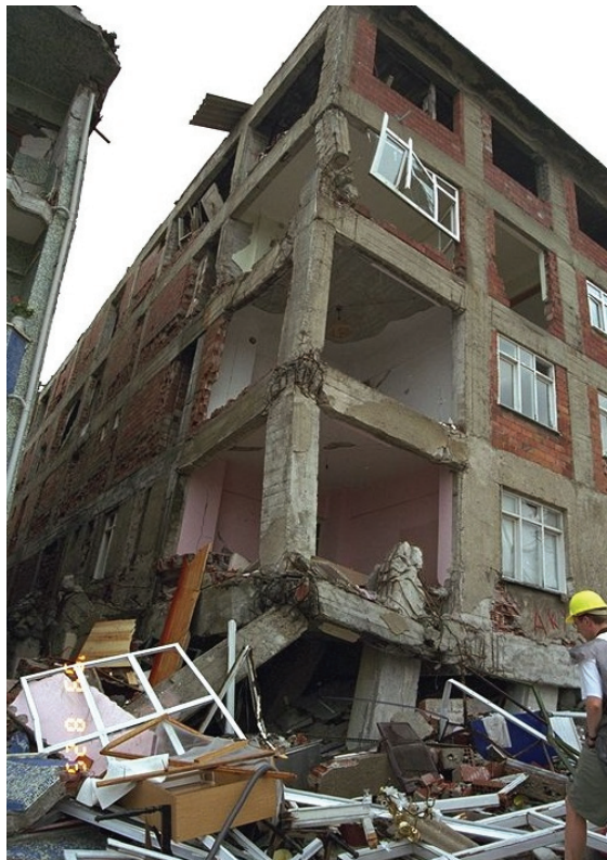
Figure 4-3 Beam-column joint failures in the 1999 Koceali (Turkey) Earthquake (Courtesy of NISEE Earthquake Engineering Online Archive).
