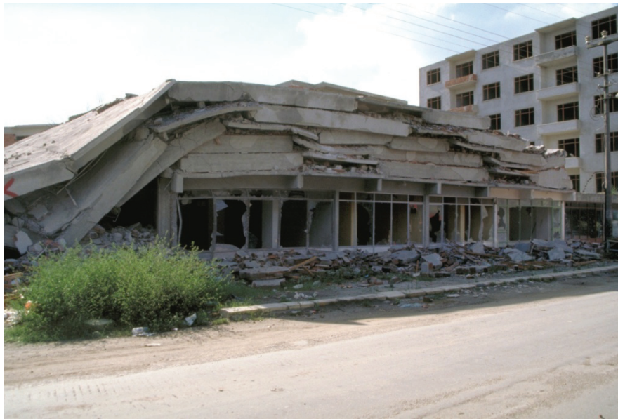
Figure 4-7 Weak frame building collapse in the 1999 Kocaeli (Turkey) Earthquake (Courtesy of NISEE Earthquake Engineering Online Archive).
