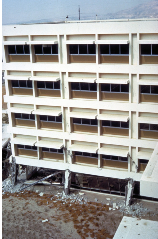
Figure 4-6 Weak-story mechanism, Olive View Hospital, 1971 San Fernando Earthquake (Courtesy of NISEE Earthquake Engineering Online Archive).
