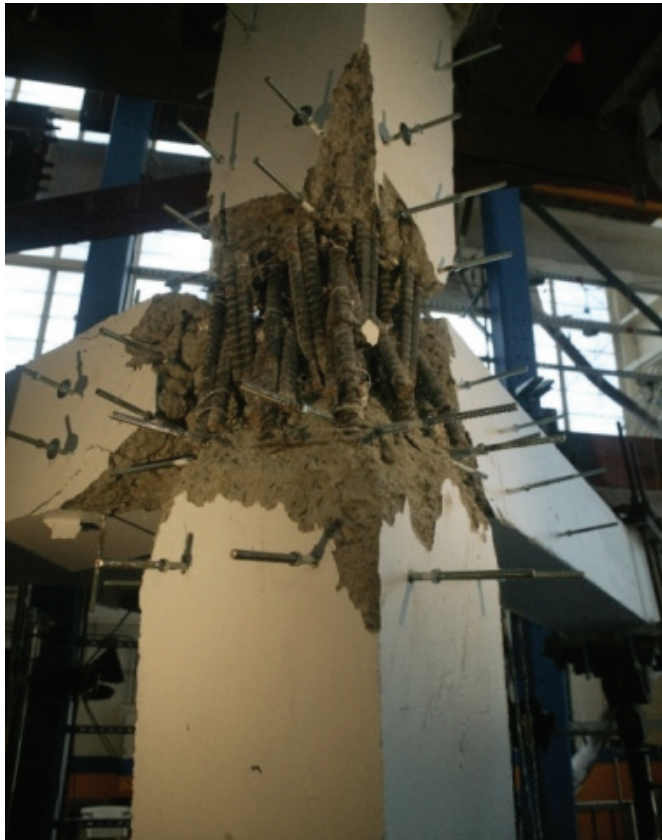
Figure 3-7 Beam-column joint specimen ID 5 tested to failure (Courtesy of NEES Grand Challenge).
