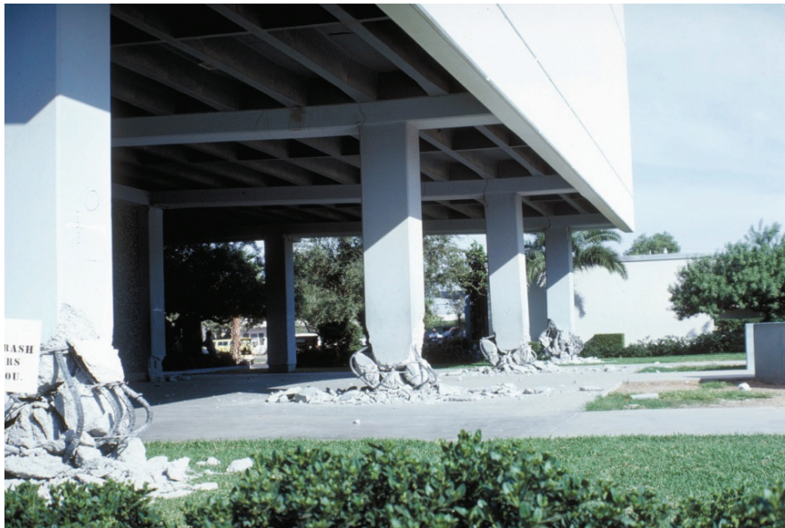
Figure 4-8 Column crushing due to discontinuous wall system, 1979 Imperial Valley Earthquake (Courtesy of NISEE Earthquake Engineering Online Archive).
