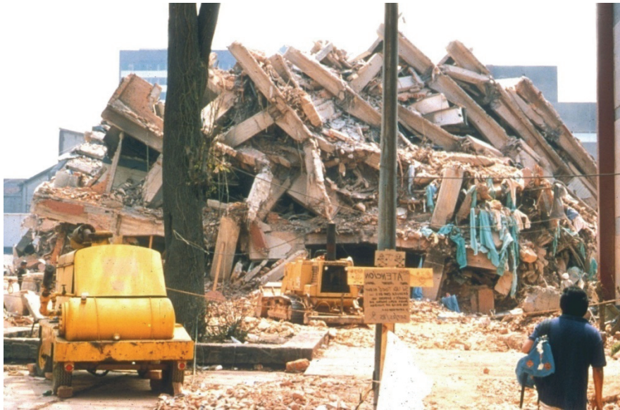
Figure 4-5 Collapse due to connection failures in the 1985 Michoacán (Mexico) Earthquake (Courtesy of Mete Sozen).
