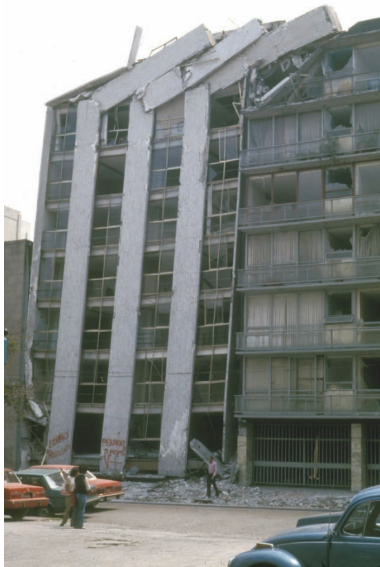
Figure 4-11 Collapse of upper stories due to building pounding in the 1985 Michoacán (Mexico) Earthquake (Courtesy of Jack Moehle).
