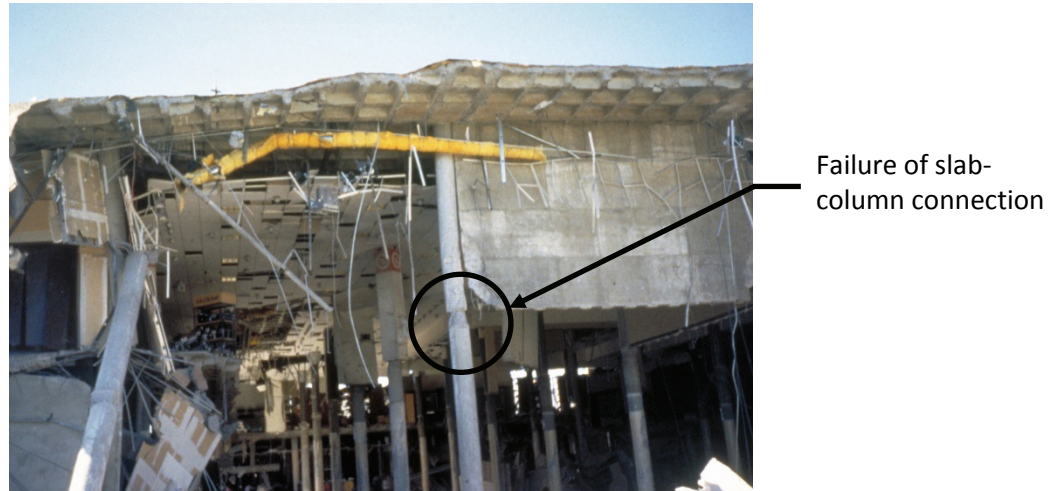
Figure 4-4 Slab-column connection failure in the 1994 Northridge Earthquake (Courtesy of NISEE Earthquake Engineering Online Archive).
