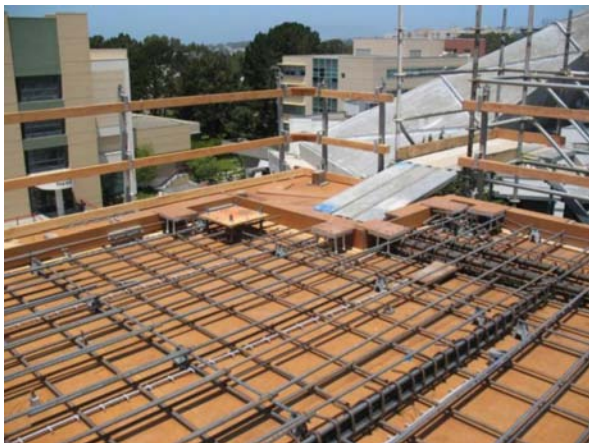
Figure 9-3 – Confinement of a collector.
