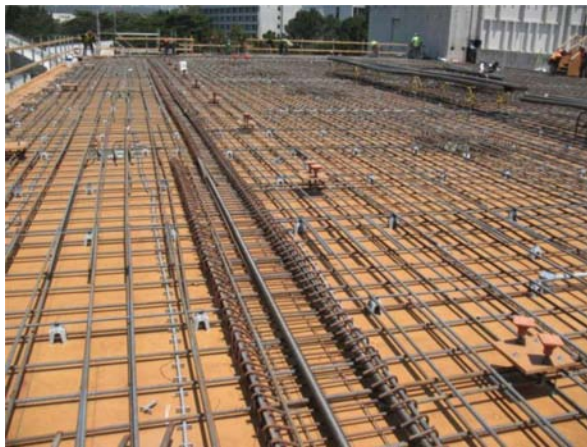
Figure 9-2 – A long collector with confinement reinforcement.
