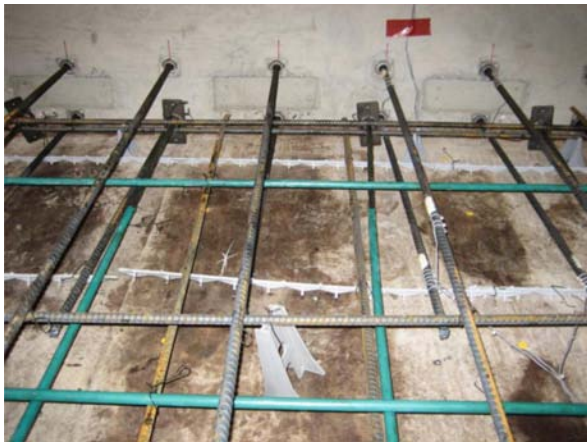
Figure 9-4 – Form savers for dowel anchorage.
