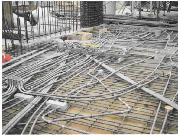
Figure 9-5 – Embedded conduit.
